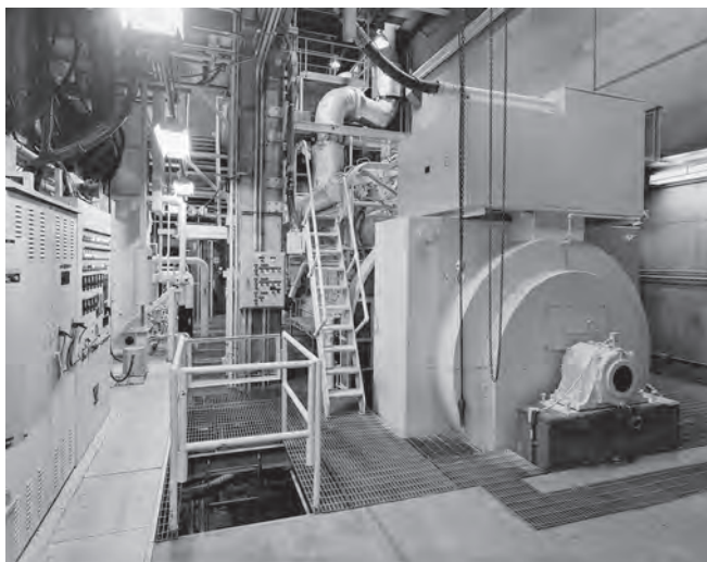
Historic view of one of the prime mover modules. This photo is actually of an identical unit in the PAR powerplant. Taken from HAER Survey document ND-9-B The generators had of course been removed when the site was decommissioned, but it was still possible to see where they were located, along with their control/switch gear. Each generator also had a ‘combustion air’ room
